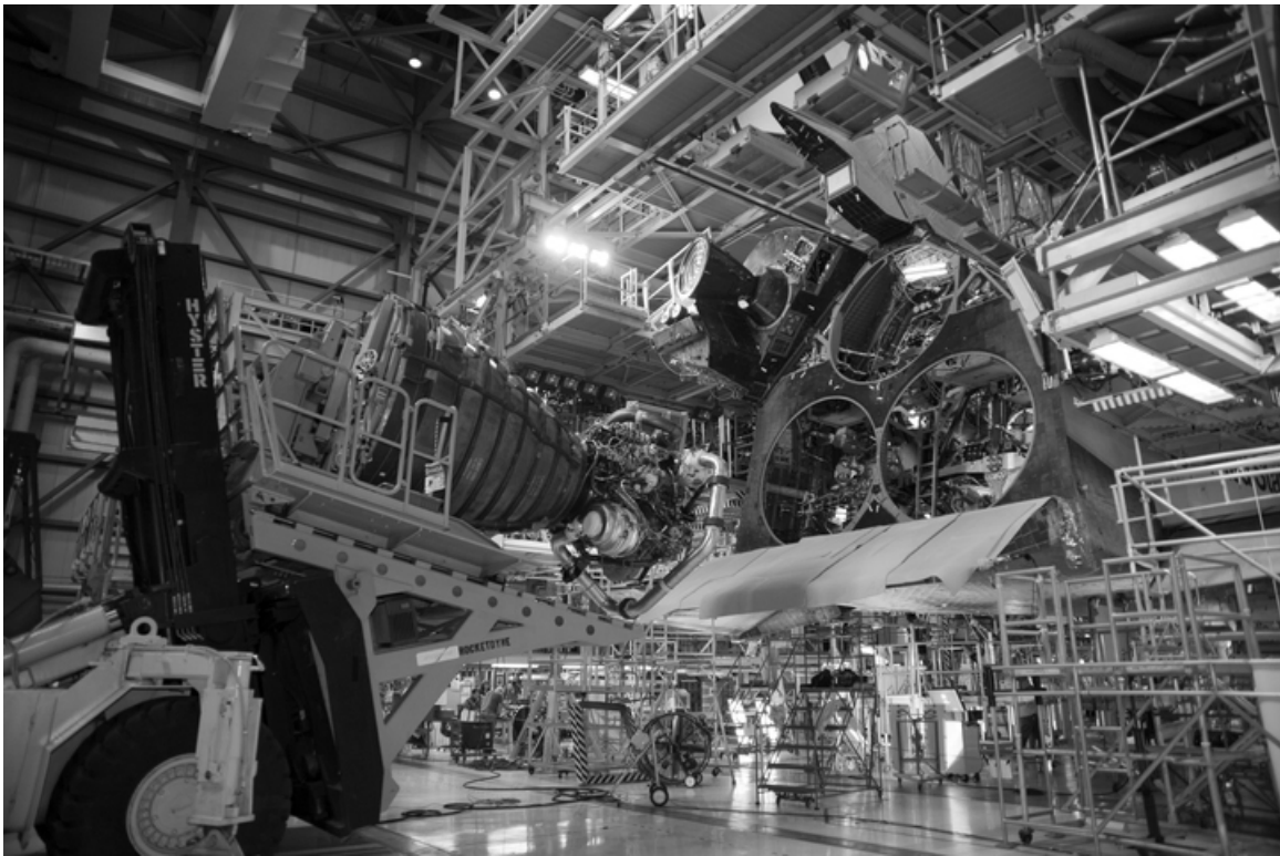
Figure C-40. Arrival of a SSME at OPF-3, Kennedy Space Center, for installation into engine position No. 1 of Discovery , camera facing northwest, June 30, 2010. Source: John F. Kennedy Space Center Online Multimedia Gallery, KSC-2010-3923.
