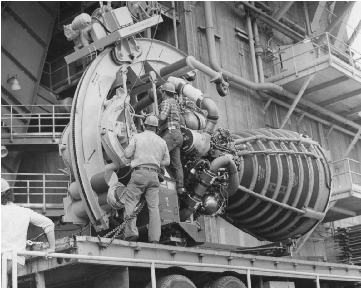
Figure C-6. Hoisting a SSME into SSC Test Stand A-2, direction unknown, 1979. Source: John C. Stennis Space Center, Stennis Image Retrieval System (SIRS), 79-116-7, accessed at http://www.ssc.nasa.gov/sirs/scripts/xmlWelcome.pl .
