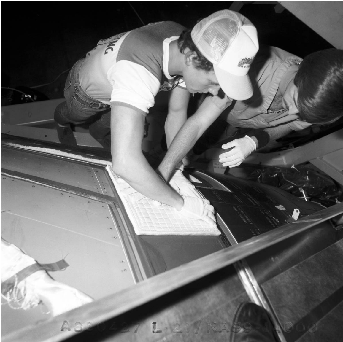
Figure B-49. Installation of AFRSI on Discovery's FRCS module in High Bay 2, AFP 42, April 27, 1983. Source: NASA, Johnson Space Center Image Repository, JSC2010-03445.
