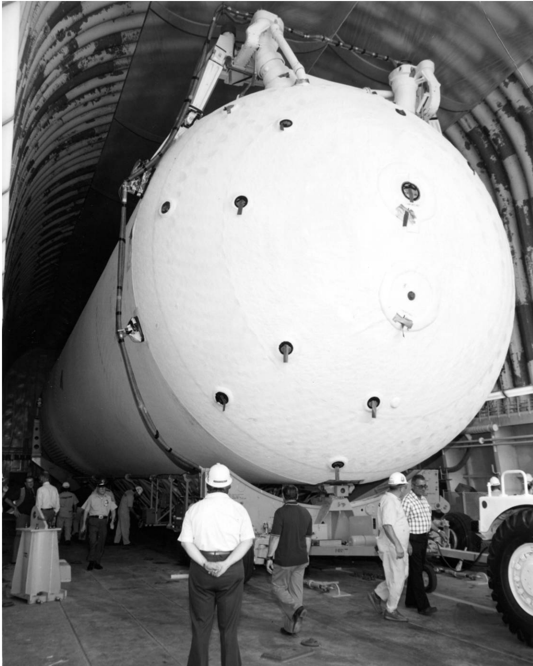
Figure D-36. ET-1 ready to be rolled into barge for 900-mile journey to KSC, June 29, 1979. Source: NASA, Johnson Space Center, Imagery Online, jsc2010e009727
