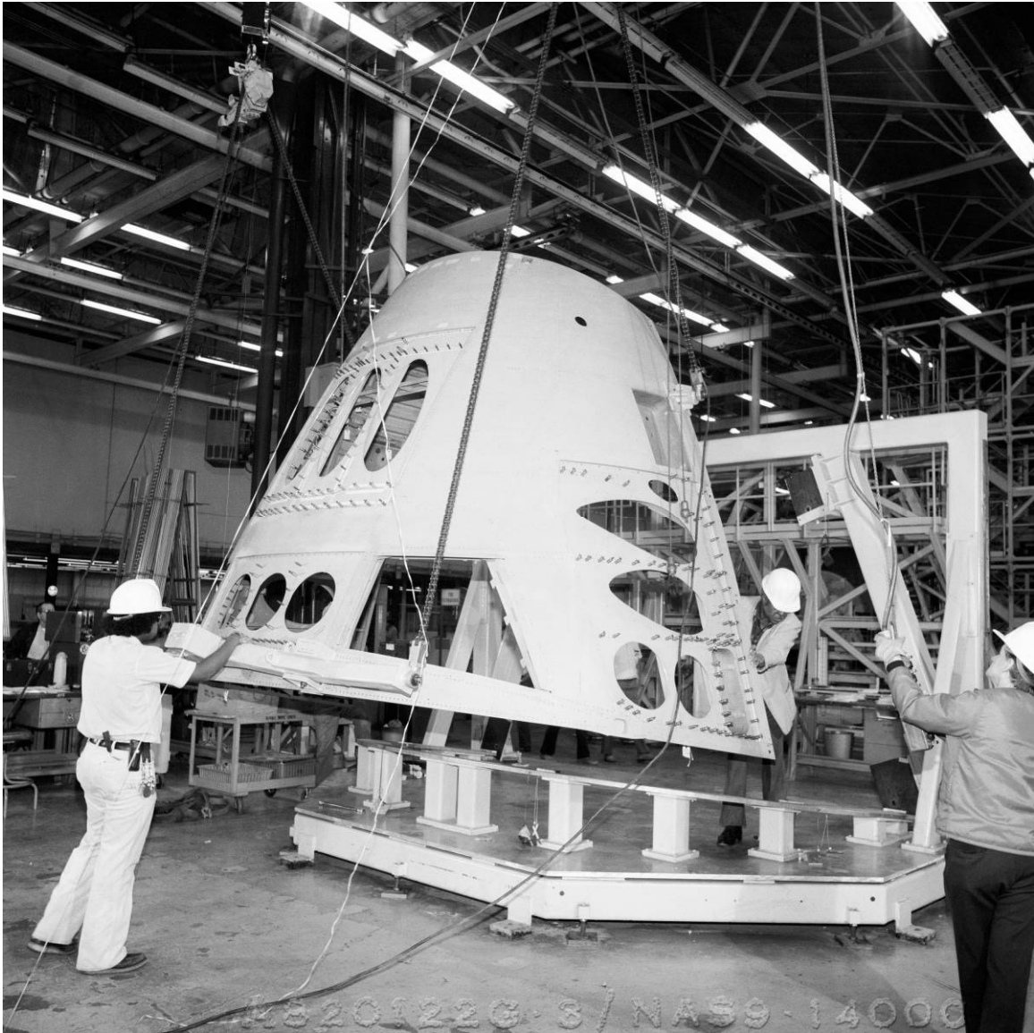
Figure B-13. Manufacturing of Discovery's FRCS module, NAR Building 1, Downey, California, January 22, 1982. Source: NASA, Johnson Space Center Image Repository, JSC2010-03228.
