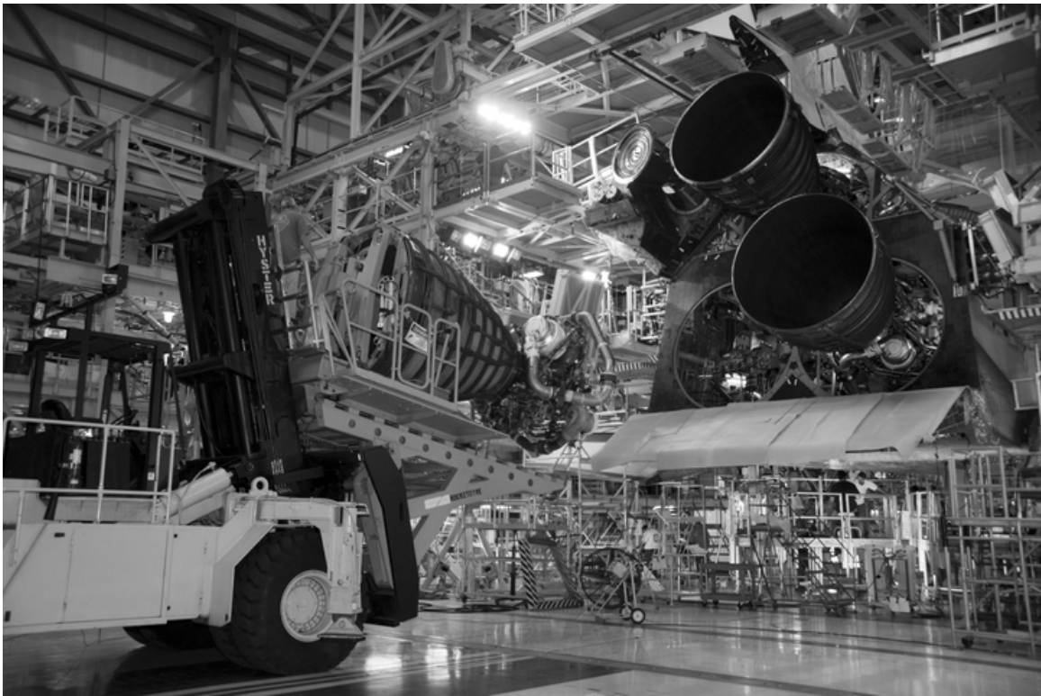
Figure C-45. A SSME being brought into OPF-3 for installation into engine position No. 2 of Discovery , camera facing northeast, July 1, 2010. Source: John F. Kennedy Space Center Online Multimedia Gallery, KSC-2010-3933.
